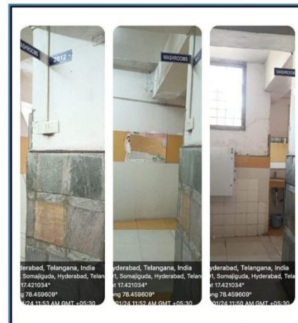
WASHROOM FACILITY IN 1ST, 2ND & 3RD FLOOR
